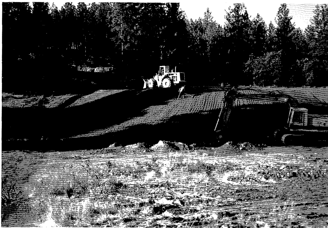
Grading of foundation layer fill material and construction of anchor trench for geomembrane liner (May 1994).
